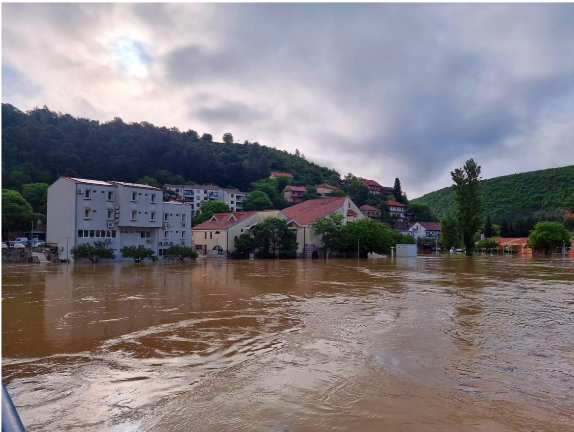
sl. 2.2.12: Pogled na zgradu Grada Obrovca, 15.5.2023. (izvor: Večernji list - https://www.vecernji.hr/media/img/43/48/7b4a77cfc3e1361ab873.jpeg )
